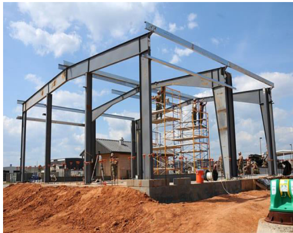
Figure 2: A pre-engineered metal building under construction
